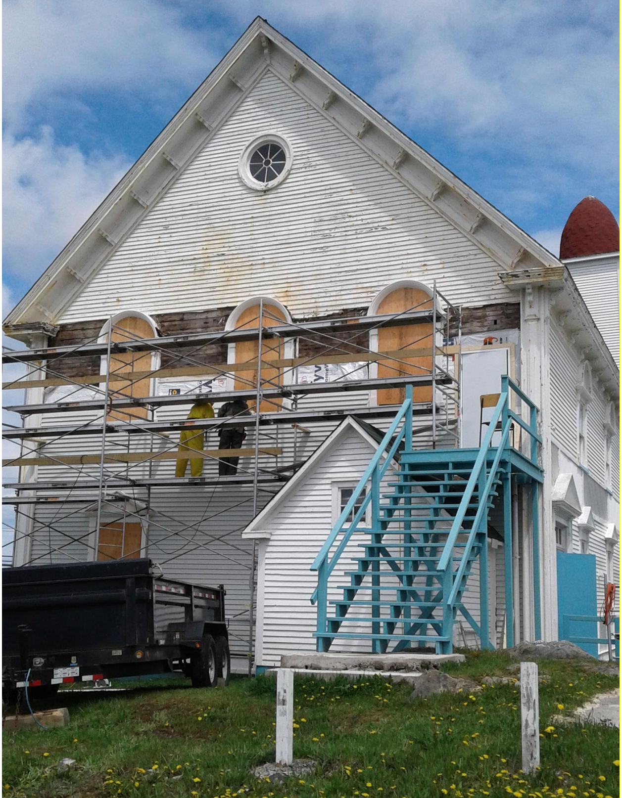
Repairing windows and clapboard on the rear of the Twillingate Masonic Lodge.
