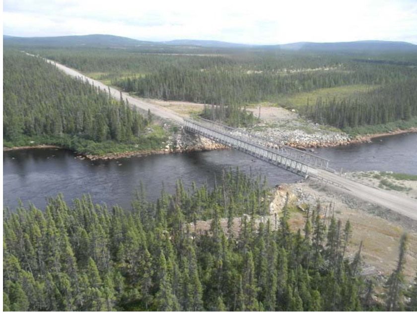
Photo 3-1 – Paradise River Bridge
