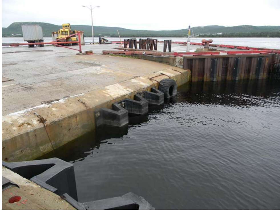
Photo 2-3 - Ferry Ramp with Fender Elements (Looking East)
