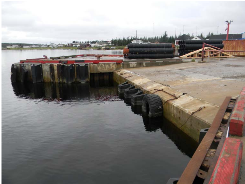
Photo 2-4 - Ferry Ramp with Fender Elements (Looking West)
