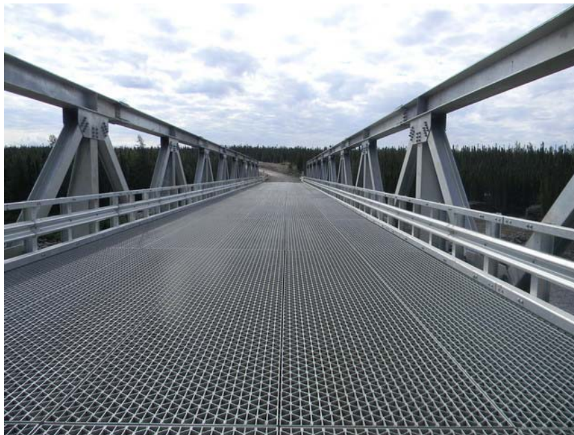
Photo 3-4: Kenamu River Bridge
