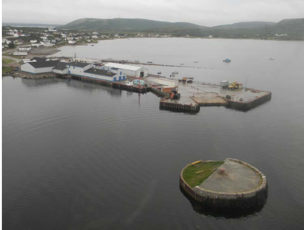
Photo 2-1 - Cartwright Facility with Wharf and Dolphin Structure
