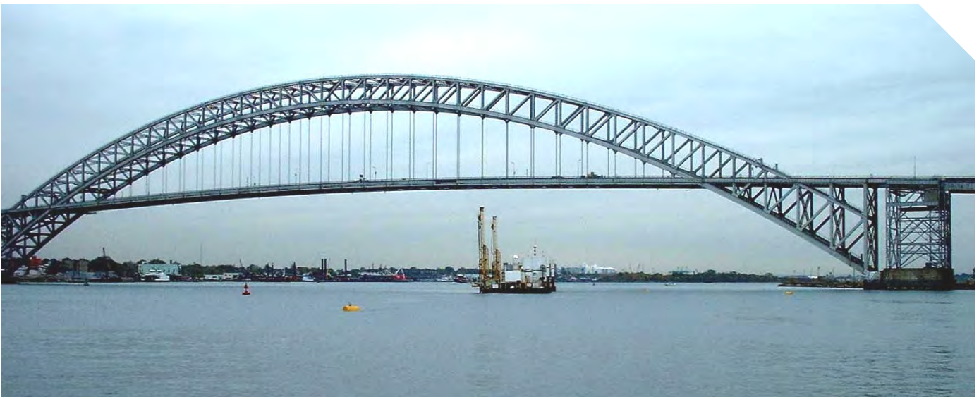
Drilling & Blasting under the Bayonne Bridge
