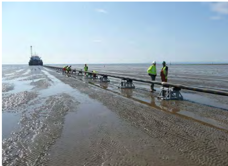
Figure 5 – Cable shore pull-in operation
