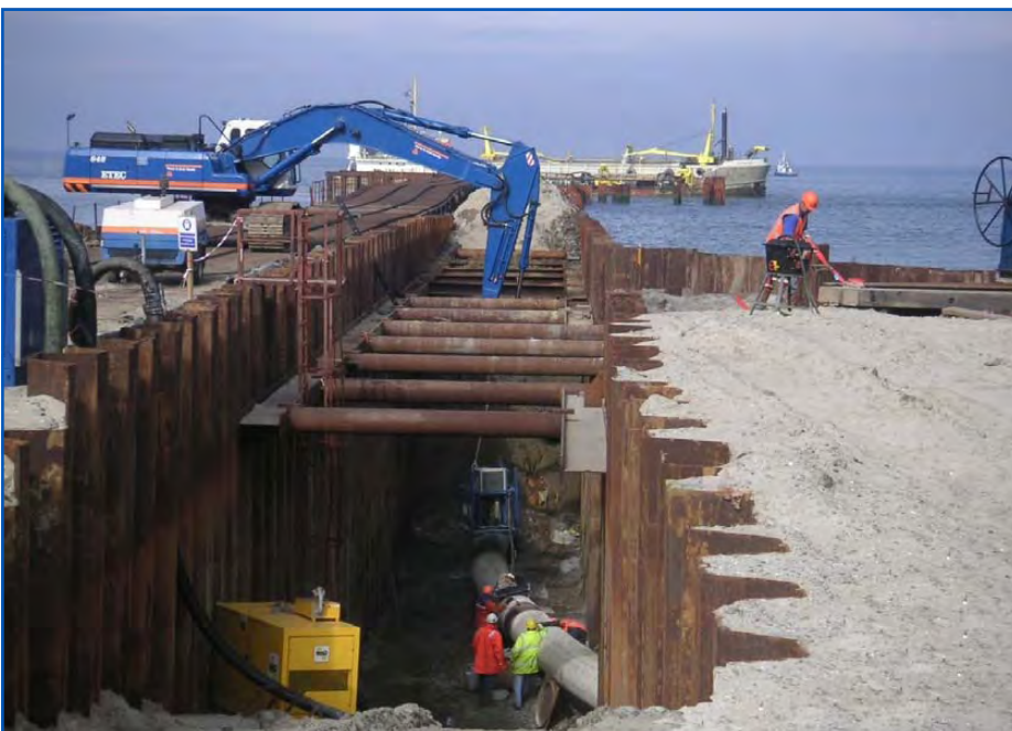
Tie-in pit and TSHD "Sospan Dau" backfilling.
