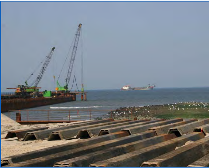
Installation of sheet piles and trenching by TSHD "Argonaut".
