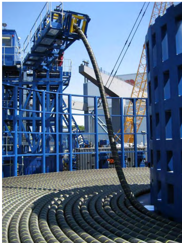
Figure 4 – Loading of Cable in a turntable
