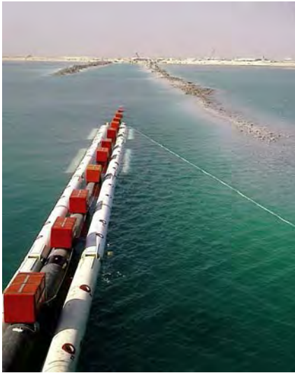
To facilitate both pull and wire installation floatation bodies were applied
