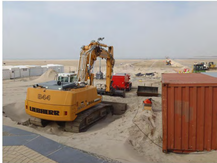
Figure 6 – Winch arrangement for Cable pull-in
