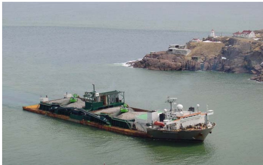
Figure 4-1 D.P. Fall Pipe Vessel "Seahorse", entering St John's Harbour
