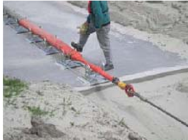
Figure 10-4 Arrival of Pullhead
