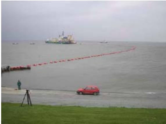
Figure 10-1 Pulling of Floating Cable
