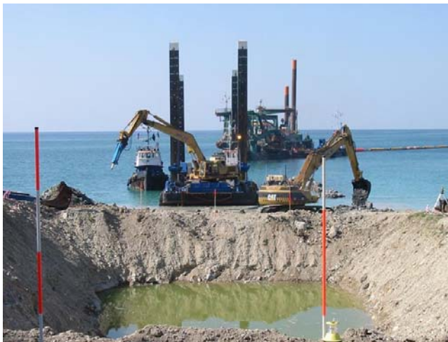
Figure 4-3 Groins from Excavated material, (Bluestream, Russian Coast)
