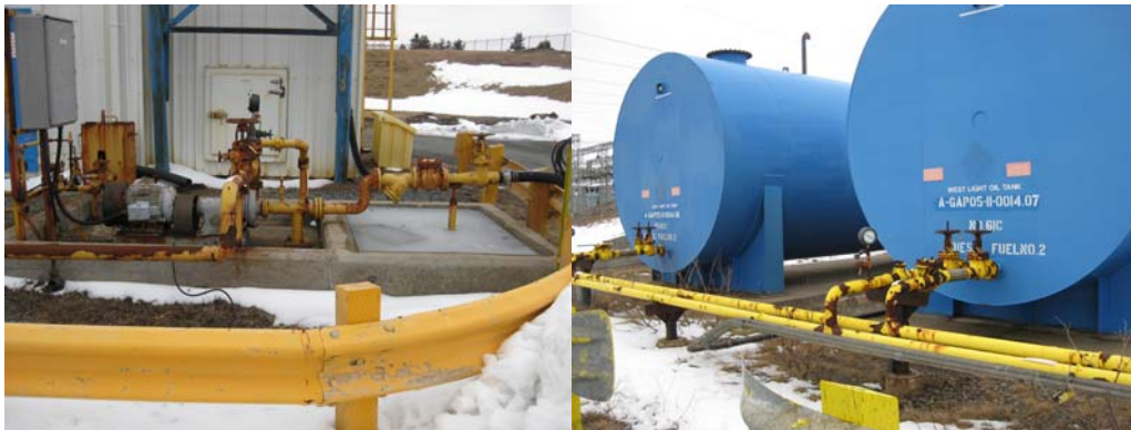
FIGURE 11-26 LIGHT OIL RECEIVING SYSTEM AND STORAGE TANKS
