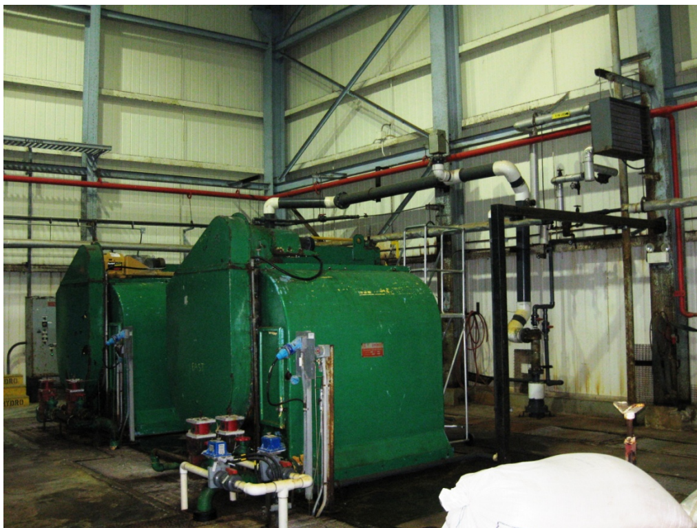
FIGURE 10-27 UNIT 3 CIRCULATING WATER TRAVELLING SCREENS
