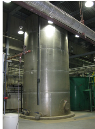
FIGURE 11-31 WATER TREATMENT PLANT – CLEARWELL AND DEMINERALIZED WATER TANK
