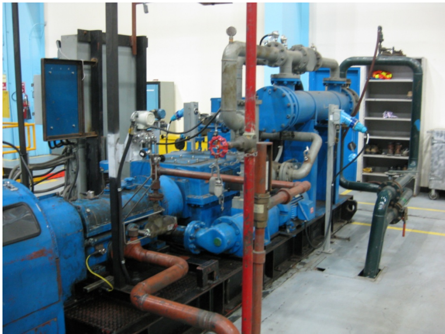
FIGURE 10-2 SYNCHRONOUS CONDENSING UNIT
