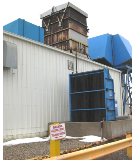
FIGURE 11-35 LIGHT OIL RECEIVING & LUBE OIL RADIATOR
