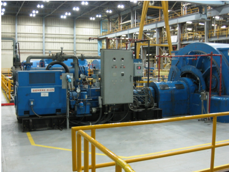
FIGURE 10-2 SYNCHRONOUS CONDENSING UNIT
