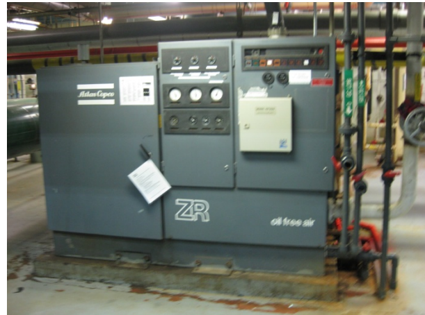
FIGURE 11-20 STAGE 1 COMPRESSOR & INSTRUMENT AIR RECEIVER
