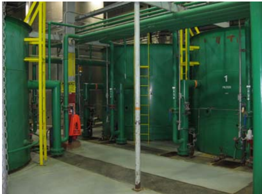
FIGURE 11-30 WATER TREATMENT PLANT – SAND FILTERS; CLARIFIER ADDITIVE TANKS
