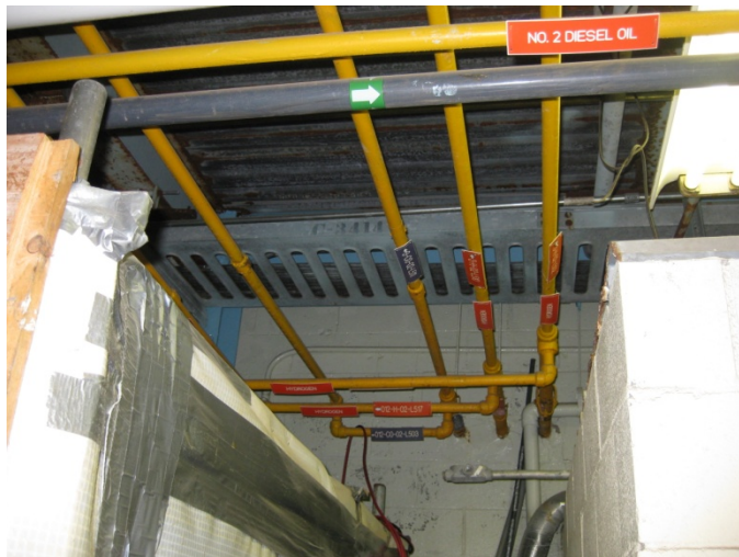
FIGURE 11-17 HYDROGEN LINES IN POWERHOUSE
