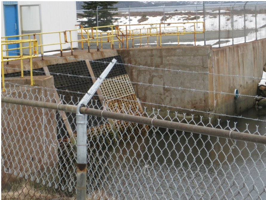
FIGURE 10-26 UNIT 3 CIRCULATING WATER INLET
