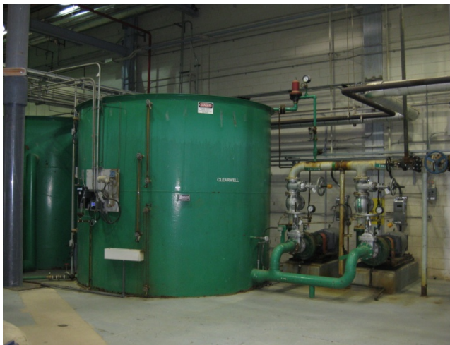
FIGURE 11-31 WATER TREATMENT PLANT – CLEARWELL AND DEMINERALIZED WATER TANK
