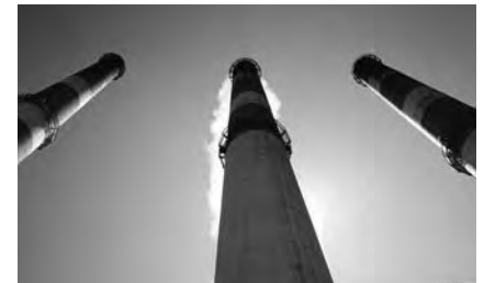
Photos above show construction of the Holyrood plant in the late 1960s. The smoke stacks of units 1 and 2 are 91m tall and the stack on unit 3 is 110m tall.
