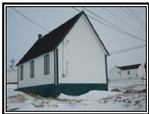
Fogo - Old School House
