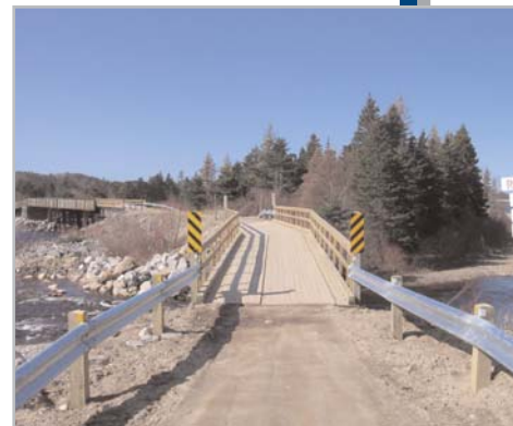
Robinsons East bridge, Dennis Tilley.
