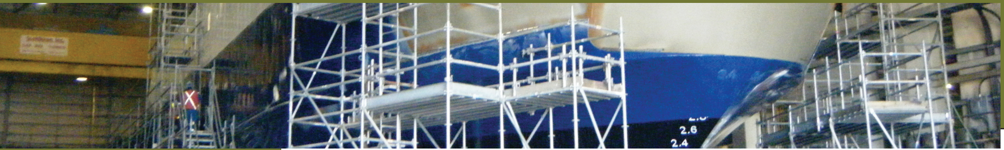
Construction of New Ferry
