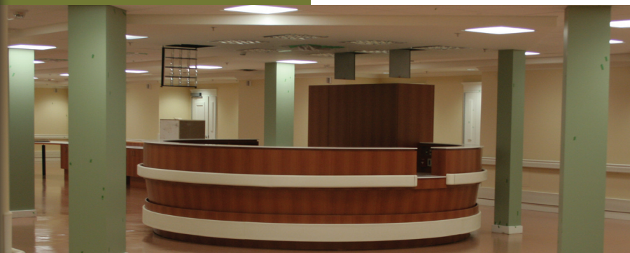
Reception Area - Corner Brook Long-Term Care Facility
