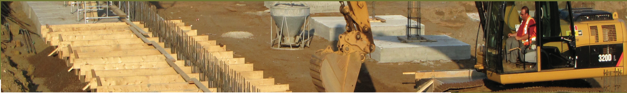
Construction of CNA - Labrador West
