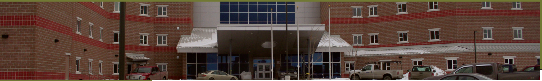
Corner Brook Long-Term Care Facility
