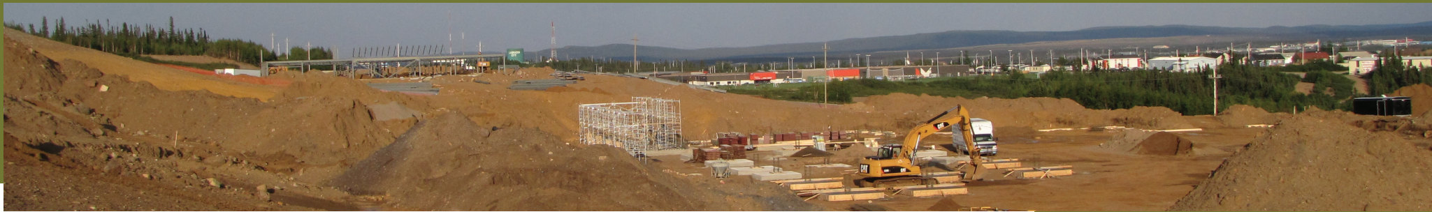
Construction of Labrador West Health Centre & College of North Atlantic
