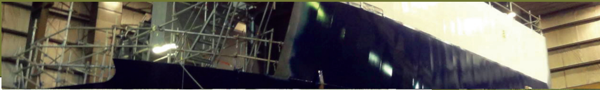
Construction of Ferry Hull 57 Bow at Marystown Ship Yard
