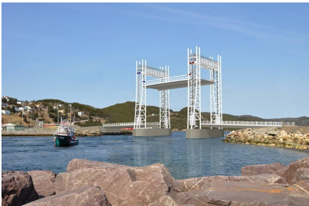
New Placentia Lift Bridge (set to open in 2016)
