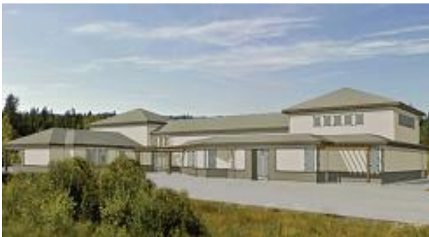
Rendition of the New Youth Treatment Centres in Paradise and Grand Falls-Windsor
