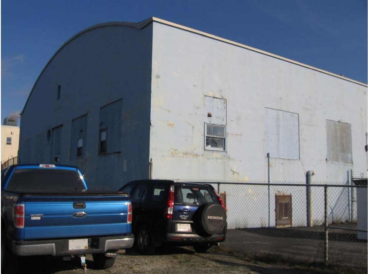
Warehouse Building 910 Pleasantville
