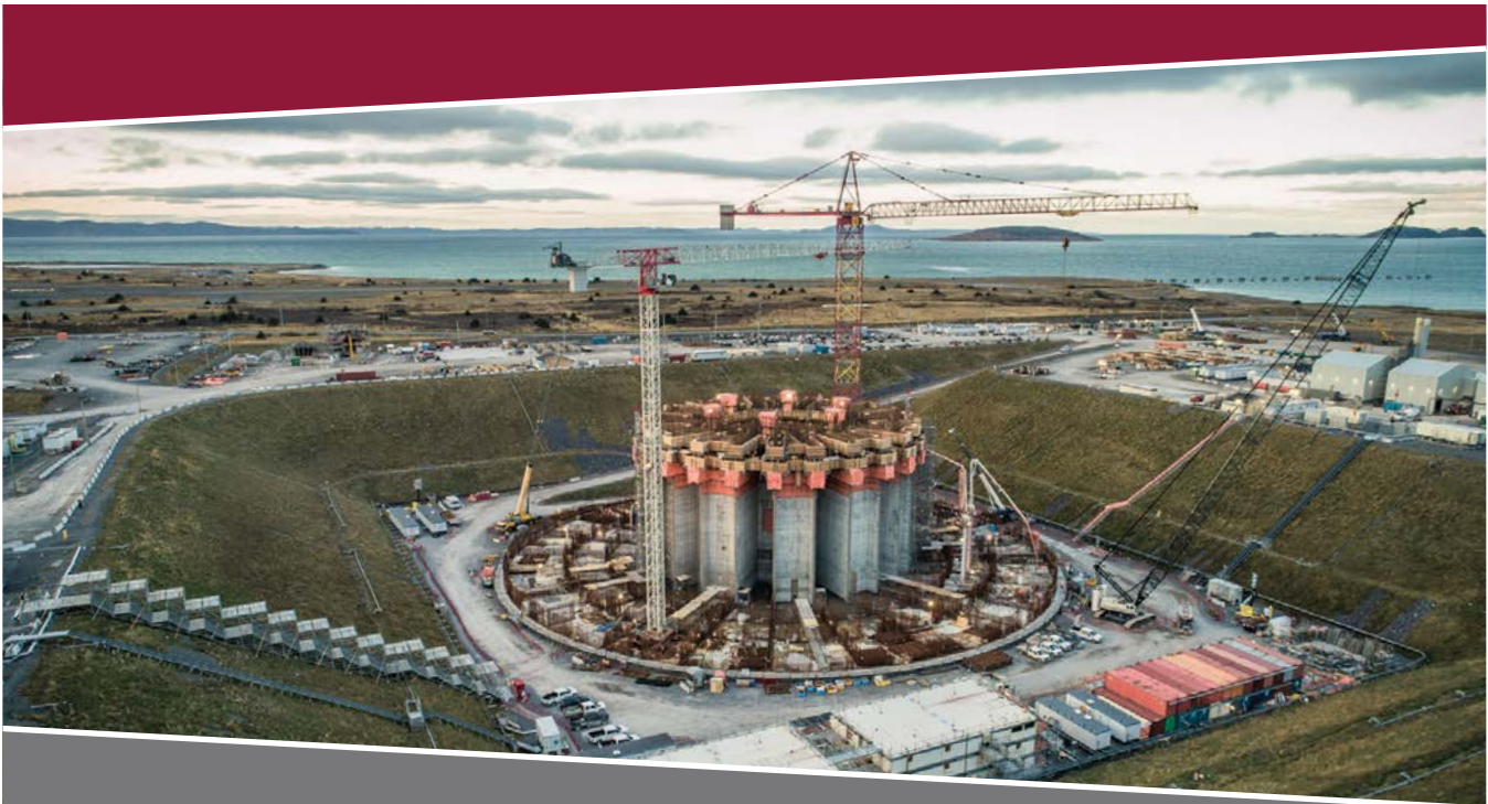
West White Rose—Concrete Gravity Structure Construction in Argentina. Courtesy: Husky Energy.
