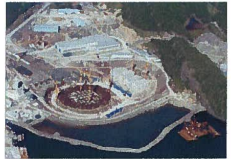
Drydock Construction and Fabrication Site
