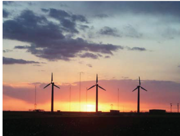
Wind power offers clean and inexpensive renewable energy.
