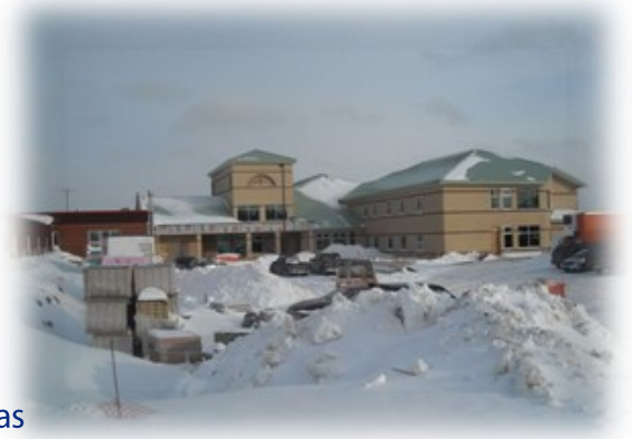
Early stages of construction of the Lewisporte District Health Centre
