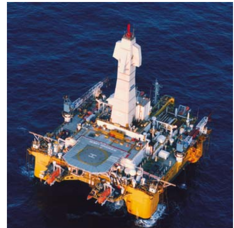
Drill Rig Henry Goodrich
