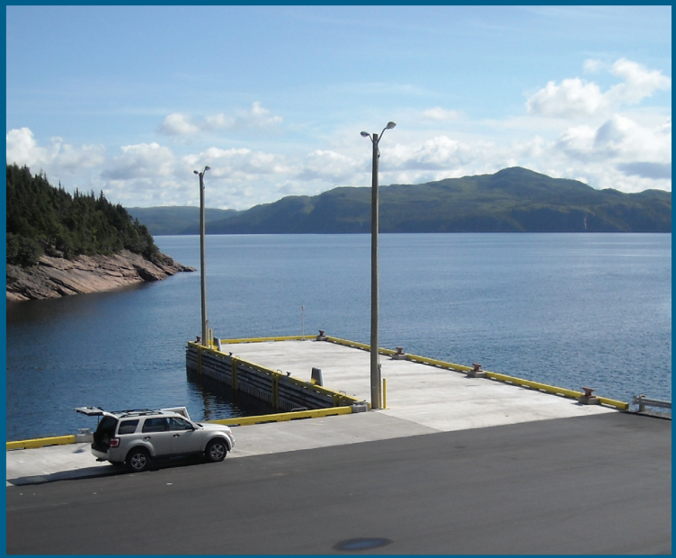
Above: the new aquaculture wharf in Pool's Cove
