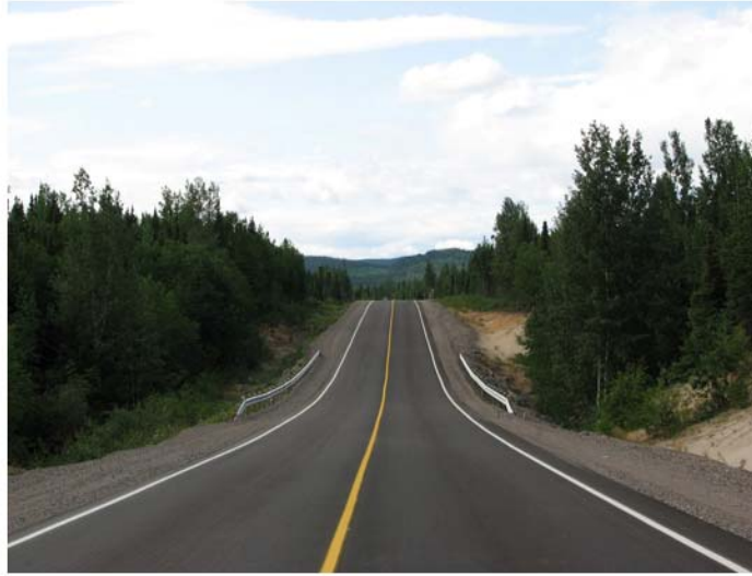
Trans Labrador Highway, Phase I
