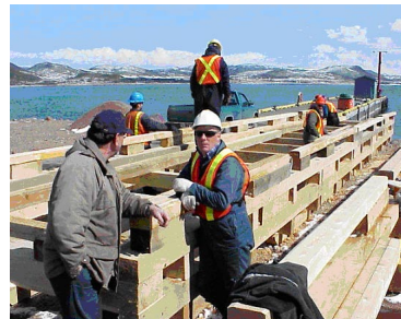
Coast of Bays, Marine Infrastructure Development
