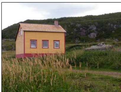
Twillingate – Jenkins House
