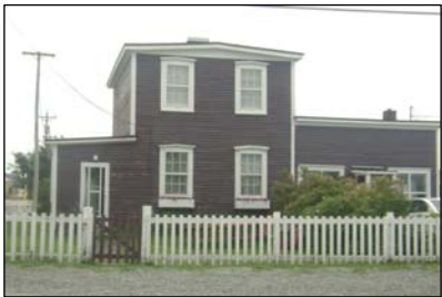
This Anglo American Telegraph Company Cable Office located in Placentia was built by Irish Merchant, Roger Sweetman in 1876. It was sold to the Anglo American Telegraph Office in New York and today is used as a private home. Original interior details have been preserved including the Telegrapher's desk in the living room.
