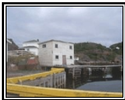
Balsom Stage - Southport Before Restoration
