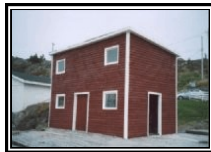
Balsom Stage - Southport After Restoration
