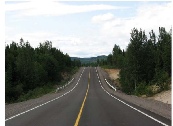
Trans Labrador Highway, Phase I
