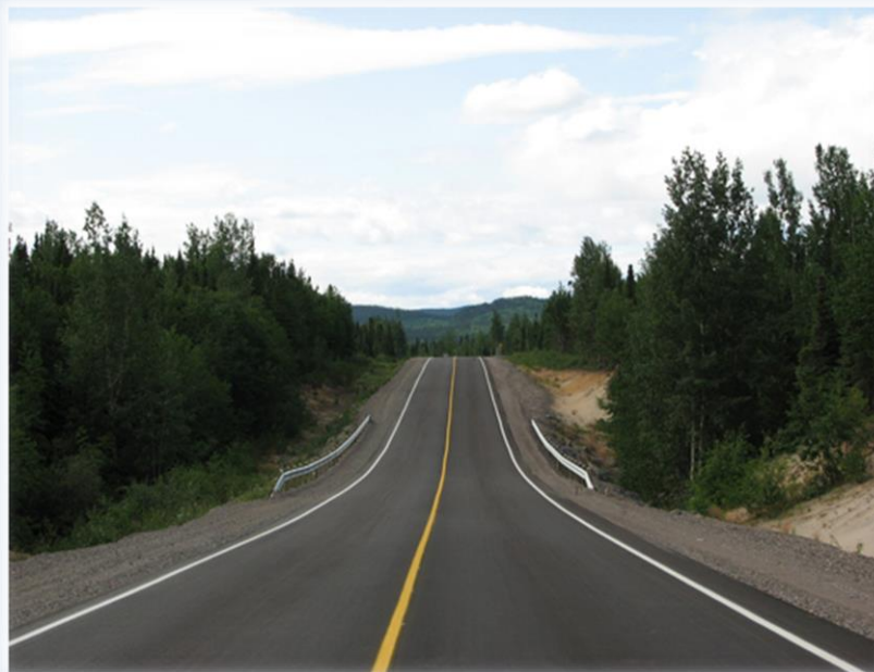
Trans Labrador Highway, Phase I
