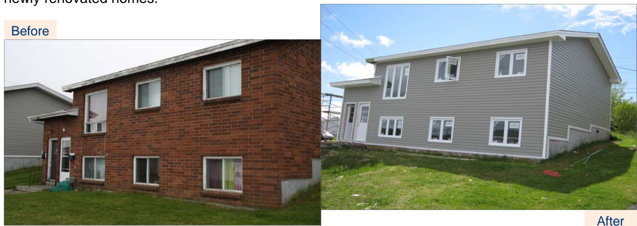
Modernization Project - Empire Avenue, St. John's
