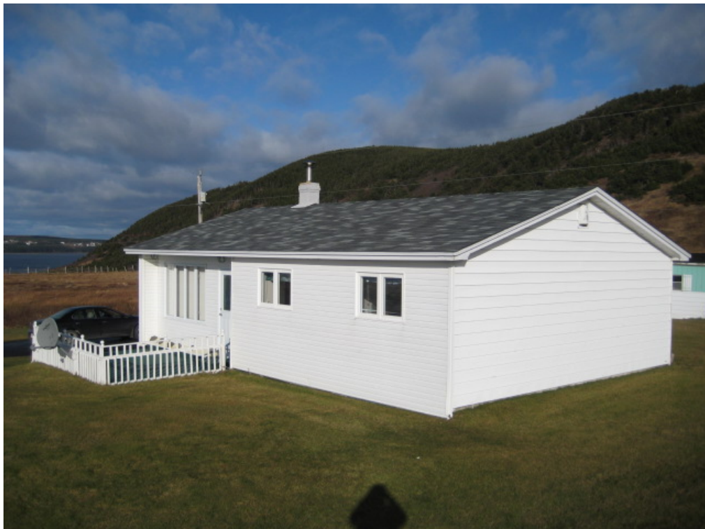
Home repaired under PHRP - St. Stephen's, NL
