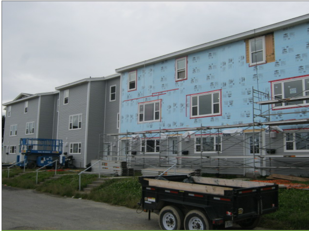
Modernization and Improvement taking place on Crestview Avenue in Corner Brook.
