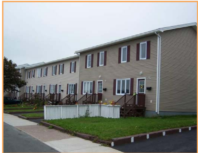
Salter Place modernization
