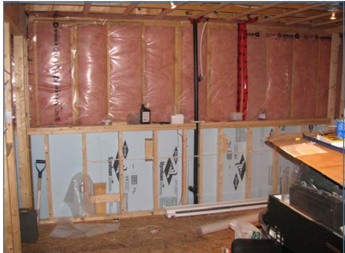
Photo by Morley Linstead, Program Delivery, NL Housing.
