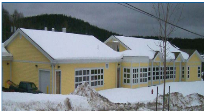
Joe Mullins Building, Corner Brook
