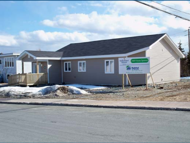
Cabot Habitat Home for Humanity Eaststaff Street. Photo provided by Wayne Lindstrom, Avalon Regional Office Maintenance.
