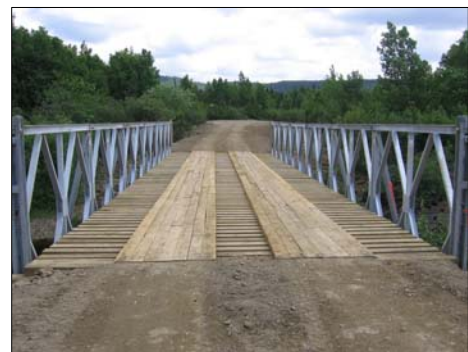
Steel Panel Bridge on a Resource Road
