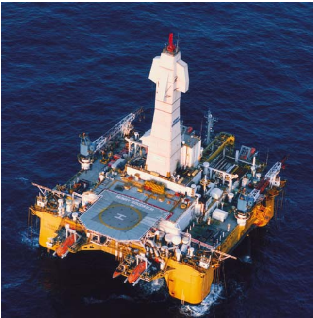
Drill Rig Henry Goodrich
