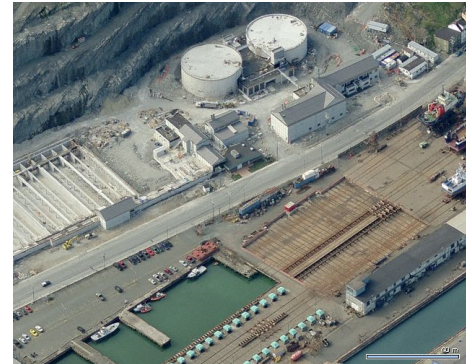
St. John's Harbour Wastewater Treatment Plant
