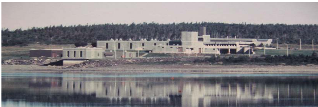
Bay Bulls Big Pond Water Treatment Plant
