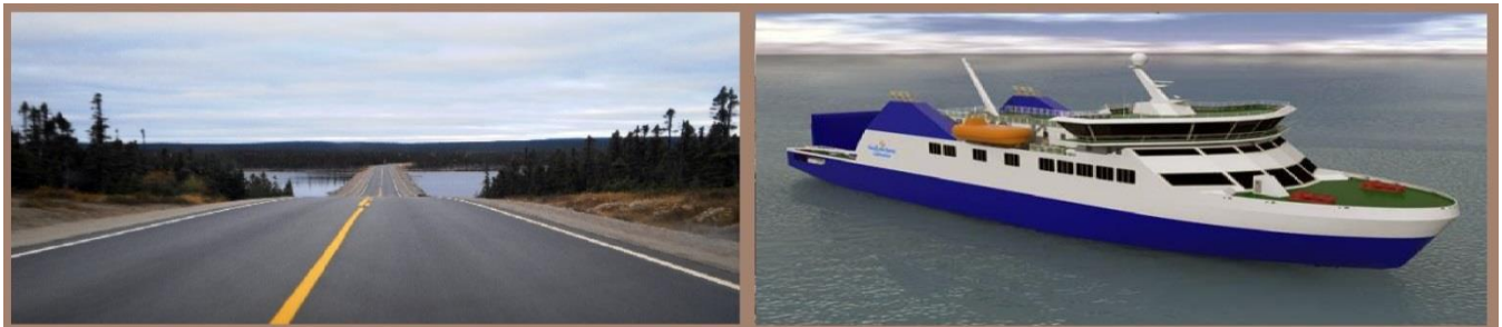
Hard surfacing of the Trans Labrador Highway, and; a rendition of a new 80-metre vessel for the provincial ferry fleet, currently under construction
