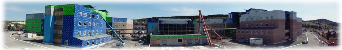
The St. John's Long-Term Health Care Facility during construction
