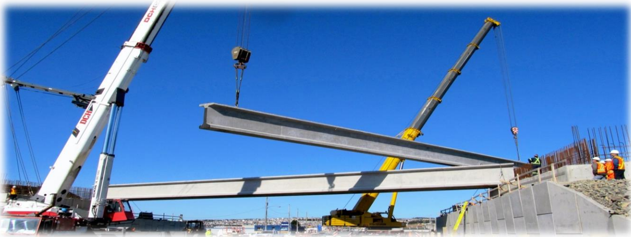
Employees constructing the Topsail Road Overpass, St. John's
