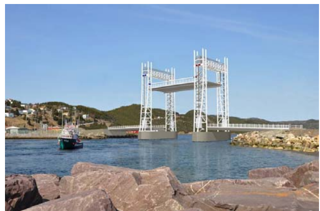
New Placentia Lift Bridge
