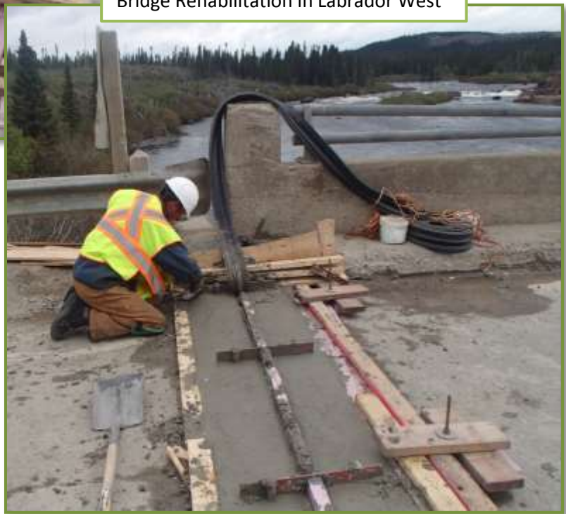
Bridge Rehabilitation in Labrador West
