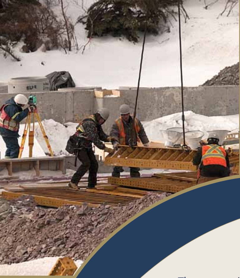
Construction workers (Dept. of Finance)
